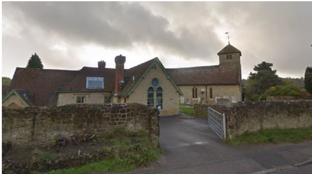
Figure 2.3- Google Street View Image showing St Bartholomew's Church (right) and The Link Building (left), viewed from Derby Road.
