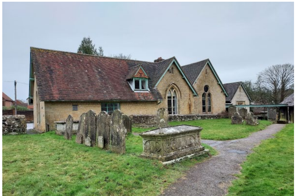
Figure 3.1 - The Link Building as viewed from the churchyard - south elevation
