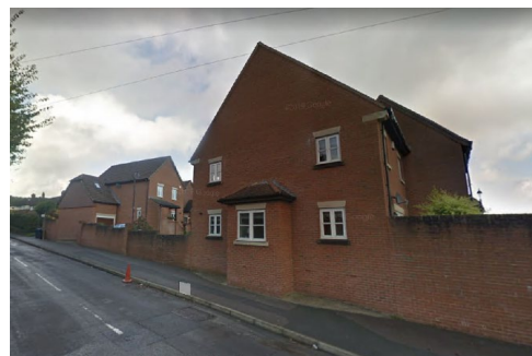
Figure 2.5 - Dwelling to the north west of the site, off High Lane.
