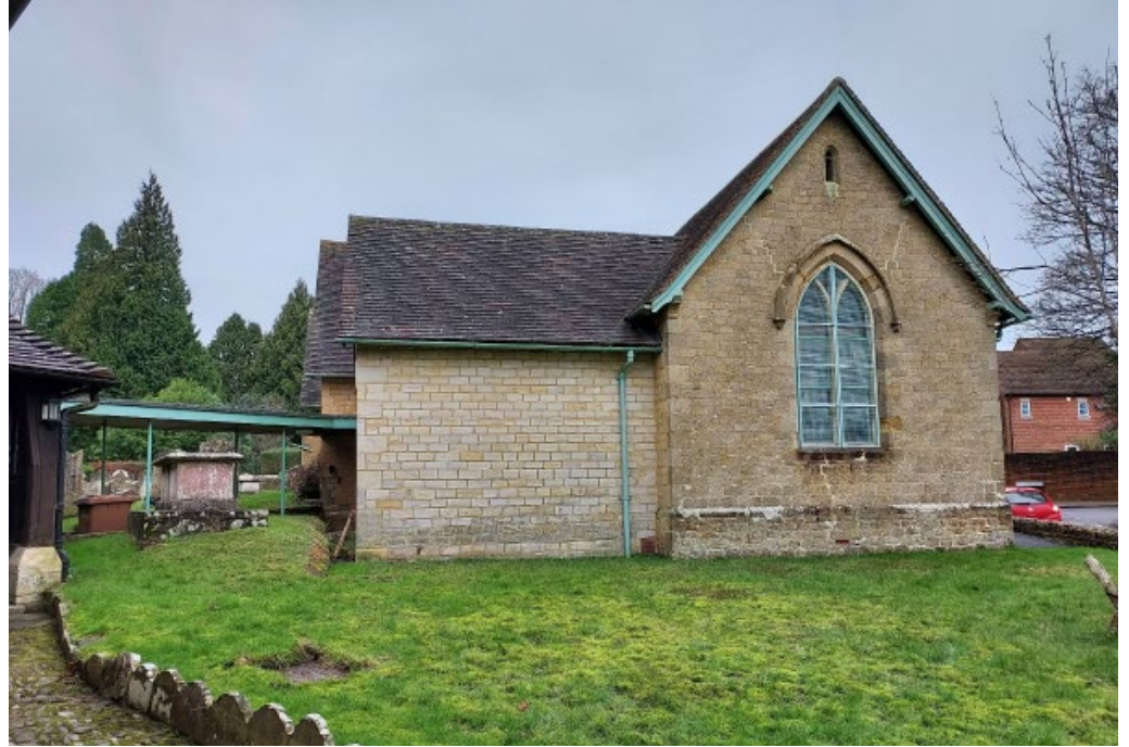
Figure 3.2 - The Link Building as viewed from Tanners Lane- east elevation
