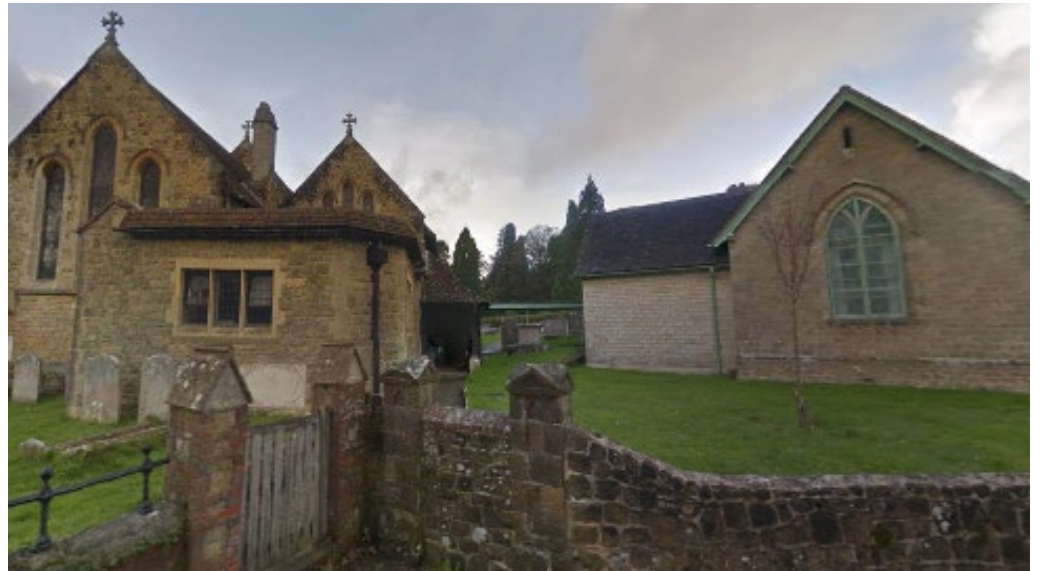
Figure 2.2- Google Street View Image showing St Bartholomew's Church (left) and The Link
